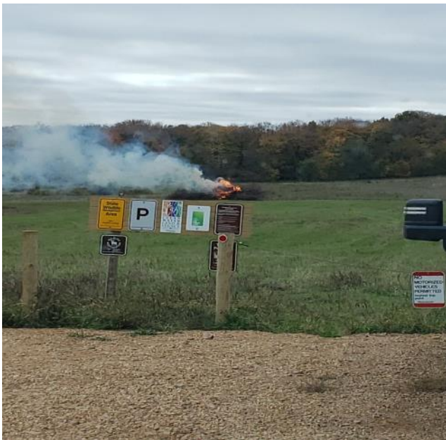
Trees and stumps were burned after removal
