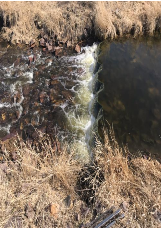
JD54 A cleaned out dam located in Cordova Township.
