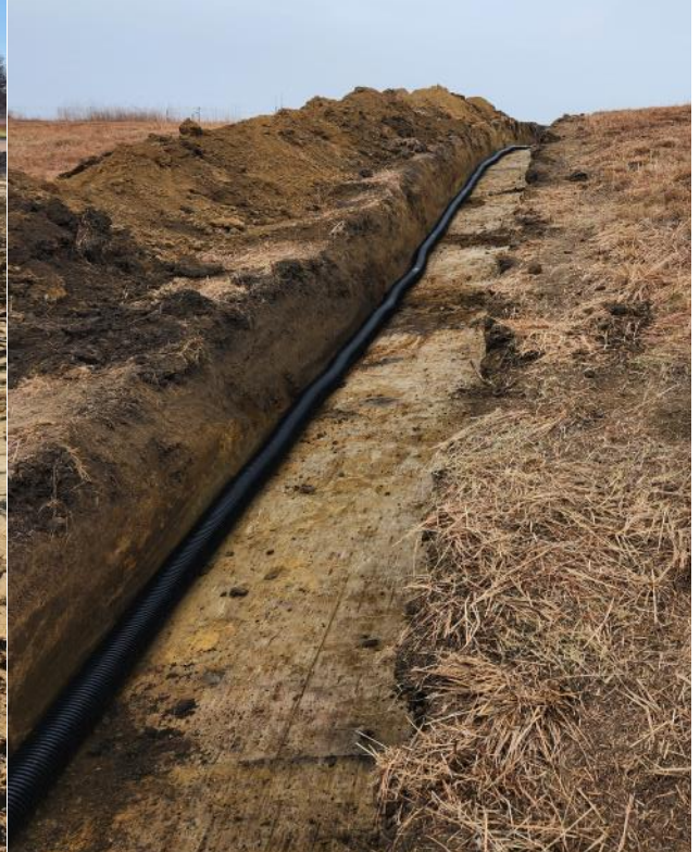
Top Left– Construction of a Farmable Sediment Basin
